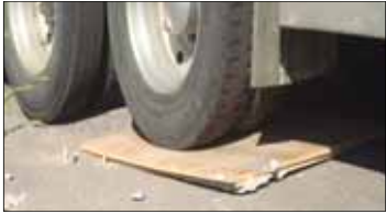
Compressive strength of the polyurethane rises as density is increased. Here, CST uses a temporary cap of double-layered plywood to contain the expansion.
